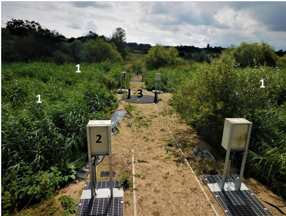
Figure 1 Gravel-Steel Slag Horizontal Flow Constructed Wetland used as a polishing step at municipal wastewater treatment plant, Devizes, Wiltshire, UK. Effective operation of treatment cells (1) is ensured by flow meters (2) synchronized with separated distribution chambers (3). (Photo. F. Bydalek)
